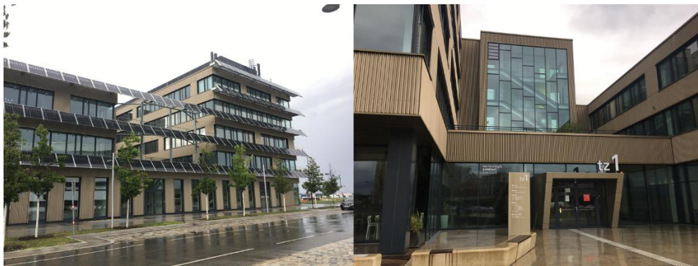
Figure 8 – View of Aspern C4 Technology Centre Building.
